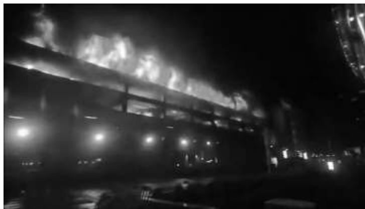
Figure 2 - Fire spread between floors via ventilation openings.
